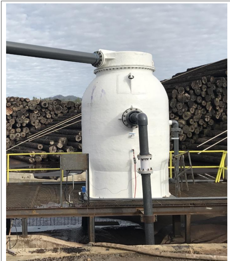
Figure 1. A 100 Cubic Foot Fiberglass HPPG filtering runoff from a lumber
