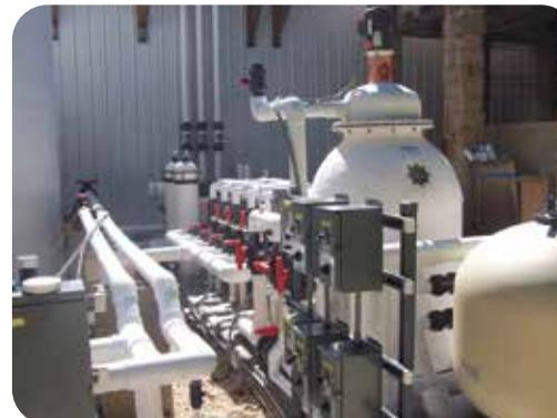
Automated PBF-10S capable of handling flows of 0.22 MGD.
