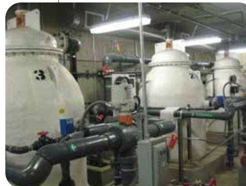
Three PBF-25S used for clarification at a flow rate of 1.6 MGD.
