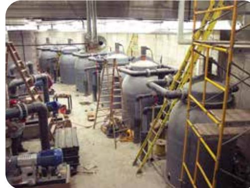
Six PBF-50S run in parallel to handle clarification for a flow of up to 6.5 MGD.
