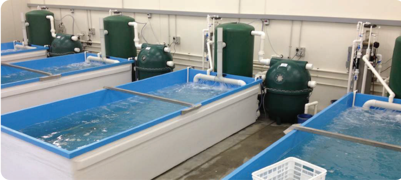
PG filters in an aquaculture facility
